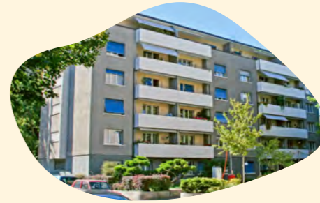
MBG Mülhauserstrasse 32–36, 40, 42 | Basel Fläche: 2'400 m 2
